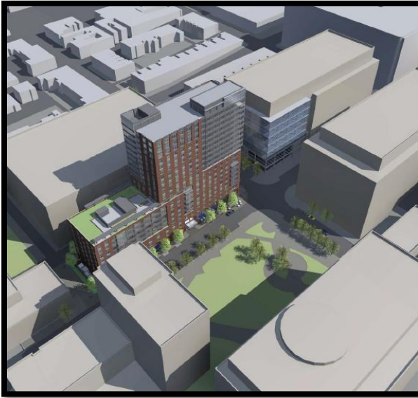
Figure 2 - an overhead showing the green roof and large green area across the street. Courtesy of Marks-Thomas Architects.
